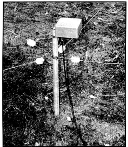
Figure 4—A photo of the central connection point at the base of a two-loop system, as installed at K9AY.
